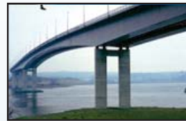
Example of a Steel Box Girder Bridge
