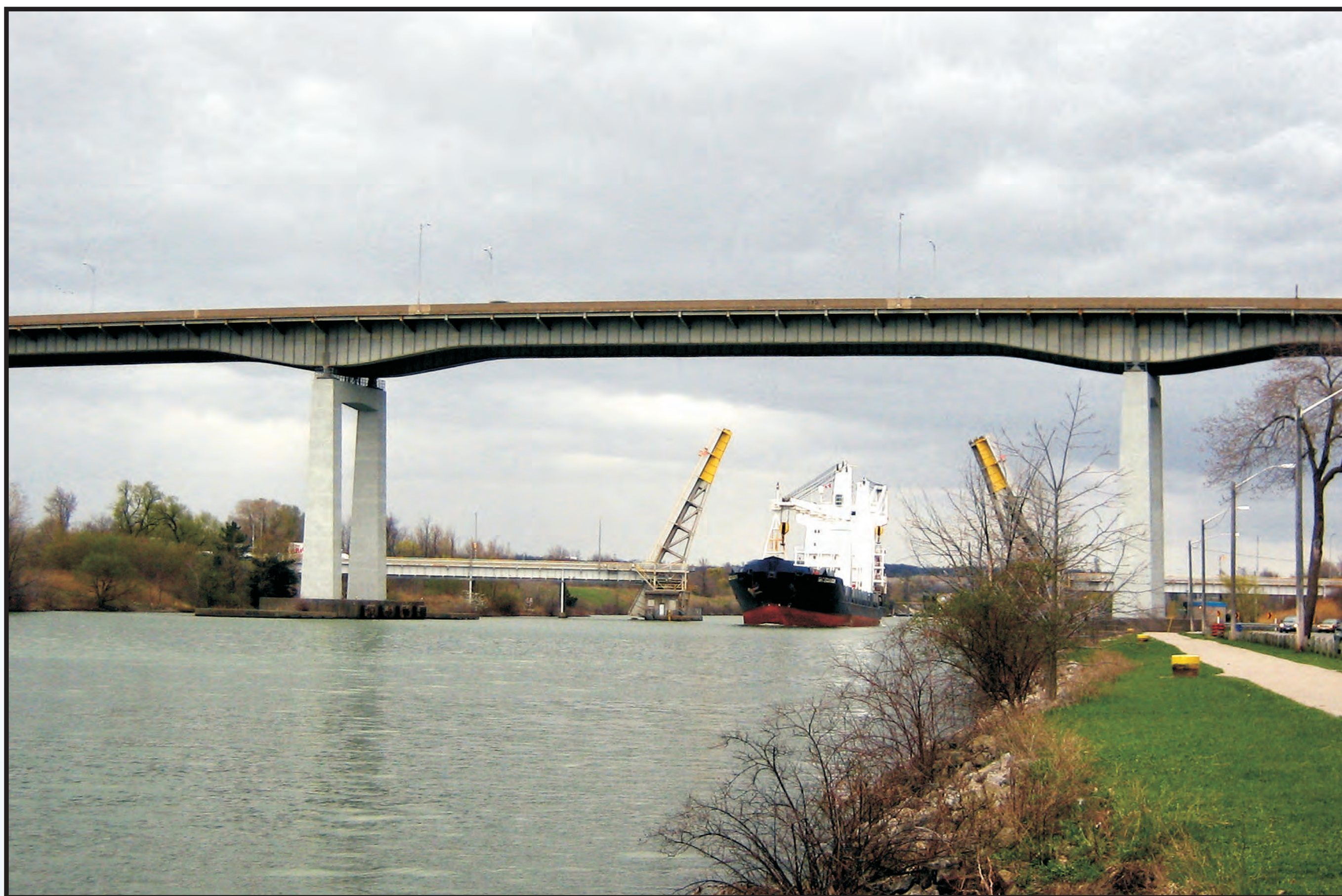
Looking south at the Garden City Skyway. In the background, a ship transits the Homer Bridge
