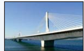
Example of an Extradosed Bridge
