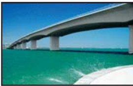
Example of a Cantilevered, Segmental Concrete Bridge
