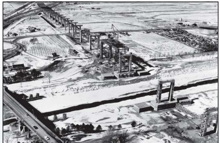
Garden City Skyway under construction in 1962, looking west.
