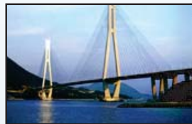
Example of a Cable-Stayed Bridge
